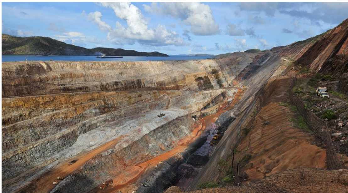
Figure 2: Koolan Island Main pit, eastern half, showing ongoing excavation of the former eastern mine haul ramp (centre) and high grade iron ore mining along the footwall (right hand side), as a loaded bulk ore vessel departs, January 2025.
